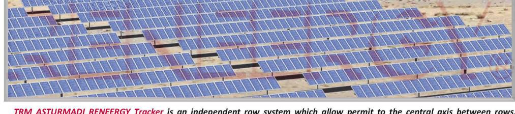
TRM ASTURMADI RENEERGY Tracker is an independent row system which allow permit to the central axis between rows, contributing to the maximum adaptability of the system to irregular local topography and on steep slopes without ground movement.
